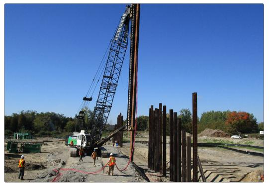
Instrumented pile being maneuvered into position
